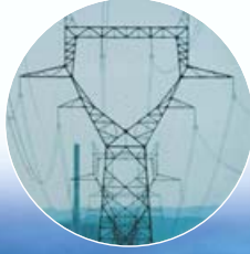
Fiber optic data cables and accessories (and OPGWs) for plant management, control and communications
